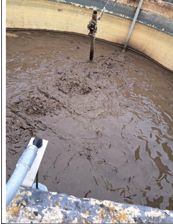
aerobic digester
