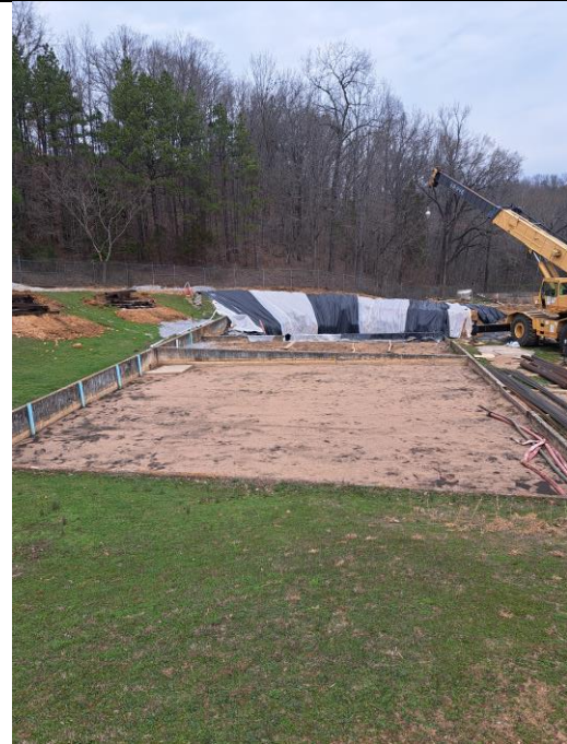
sludge drying beds (the one on the right has not been used for several months)
