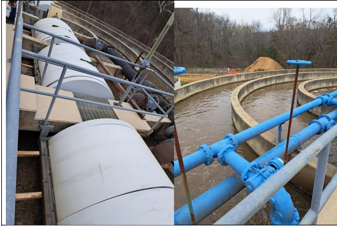
oxidation ditch
